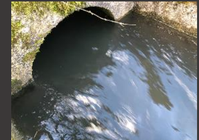
Storm tank discharge at STW Outfall
