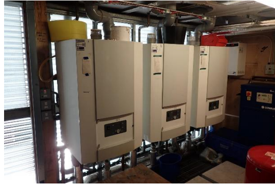
Figure 43: Heating Boilers.
