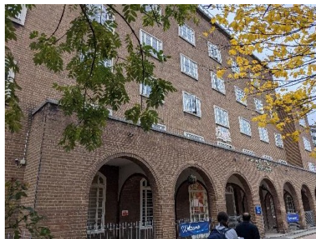
Figure 49: Floyer House Front of Building.
