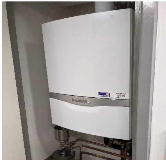
Figure 29: Condensing Boiler.
