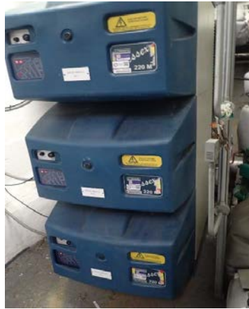
Figure 47: Modular Boiler.
