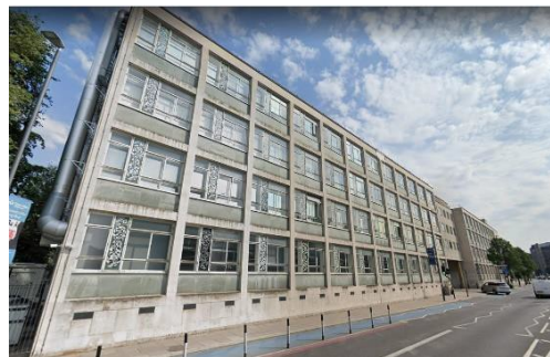
Figure 16: Mile End Road Façade.
