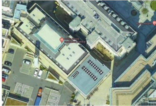
Figure 77: Robin Brook with adjacent New Energy Centre.
